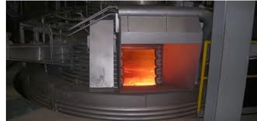
b) open door of the ladle furnace
