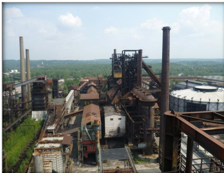
Fig. 13 (Cowper) heat blower and blast furnace.
