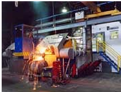
Fig. 11.2 Induction medium-frequency melting furnace for melting grey cast iron, Roučka Slévárna, a.s.
